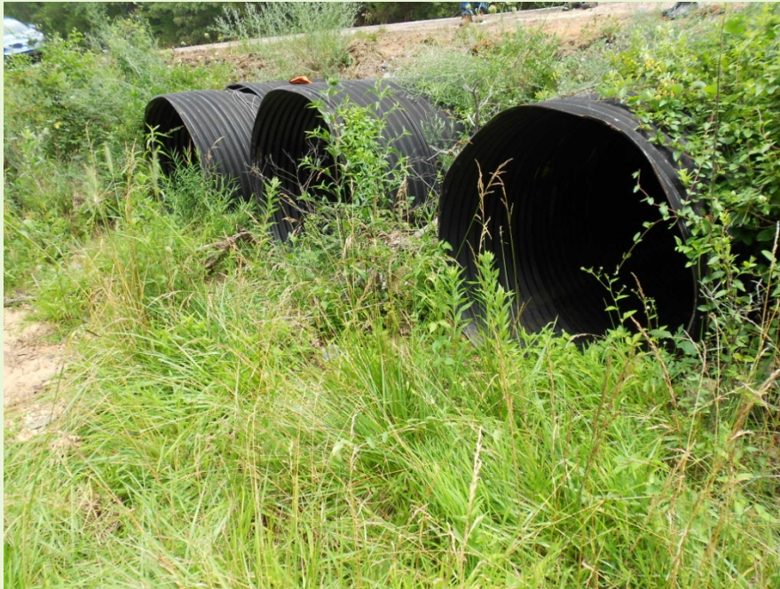
Figure 6. Exposed ends of the pipes in Arkansas
