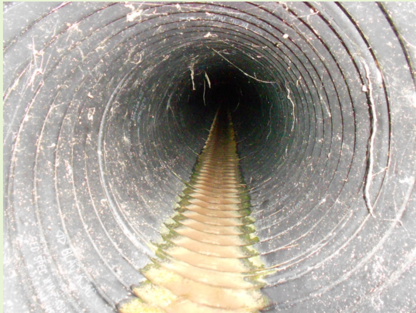
Figure 15. Typical good conditions of the polymer coating
