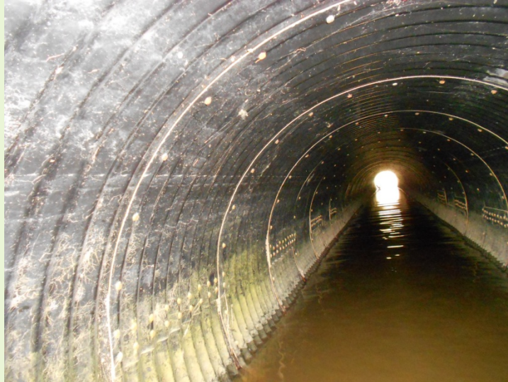
Figure 13. Typical good conditions of the polymer coating
