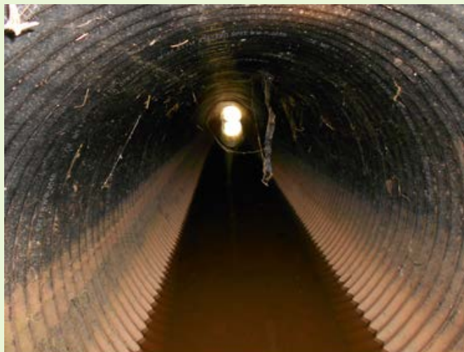
Figure 17. Example of polymer in good condition in Rapides Parish
