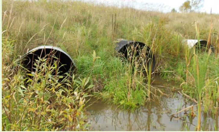
Figure 11. Pipes side-by-side under Hantz Rd.
