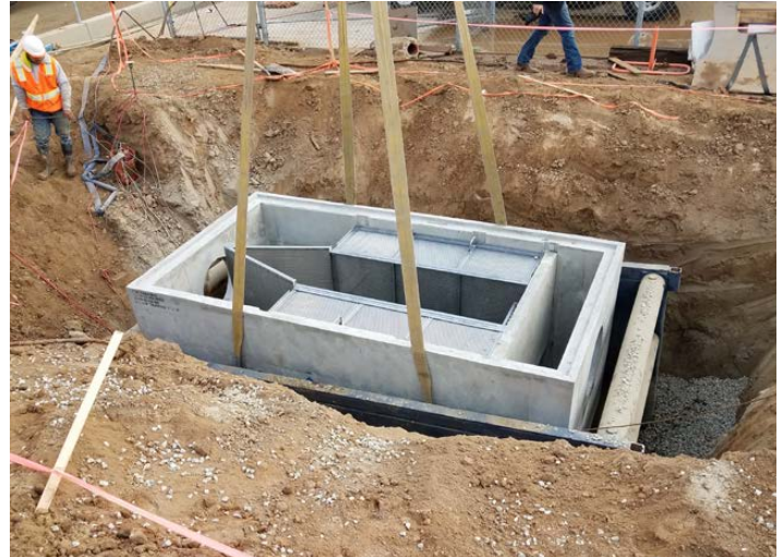
Internal components are installed prior to delivery, reducing installation time.
