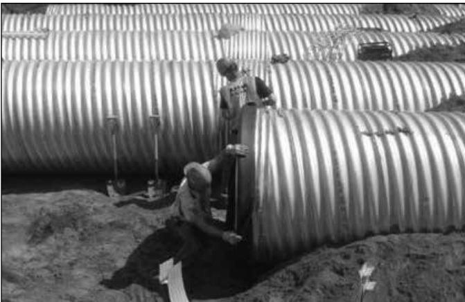
Placement of flat neoprene basket on end of CMP
