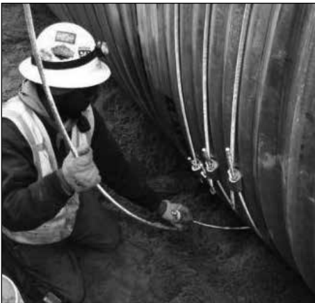
Some jobs may require special bands, such as rod and lug connection, flat bands, or dimple bands.
