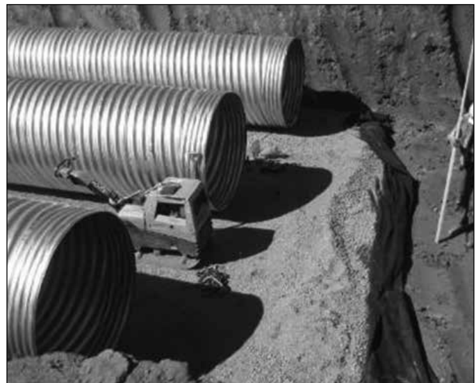
Culvert foundation required undercutting and importing 18" of granular fill for pipe bedding.
