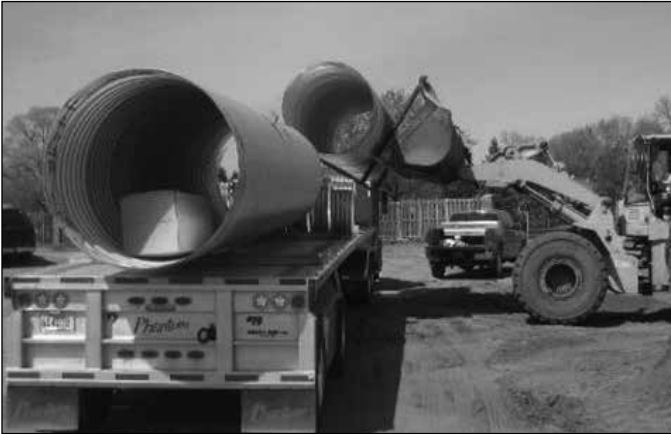
Lifting CMP off the flatbed with a front end loader and forks
