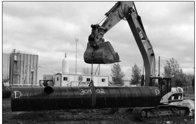
Lifting polymer-coated CMP with nylon straps
