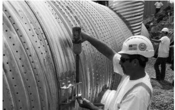
Tightening bolts on a corrugated band.
