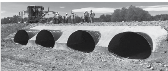
Examples of Multi-Barrel CMP Culverts
