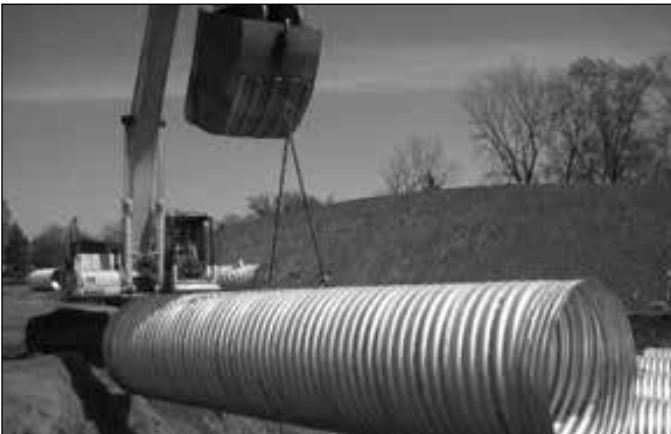
Lifting CMP utilizing factory attached lifting lugs
