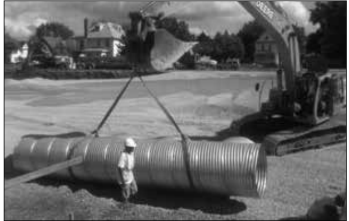
Lifting Aluminized Type 2 (ALT2) CMP with nylon slings
