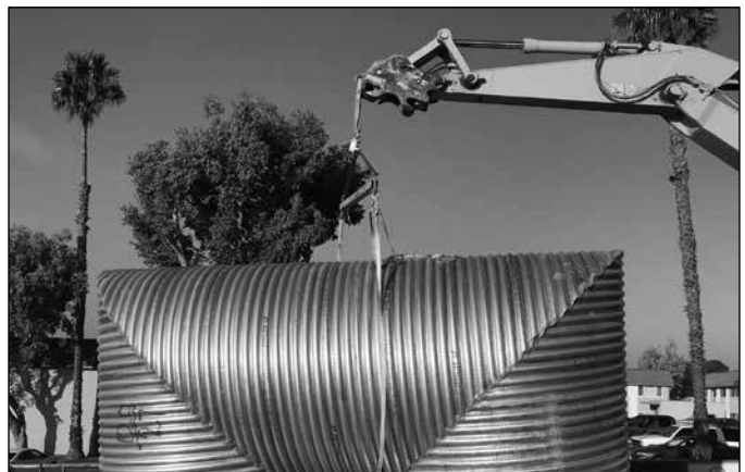
Spreader bar used to lift CMP custom fitting.
