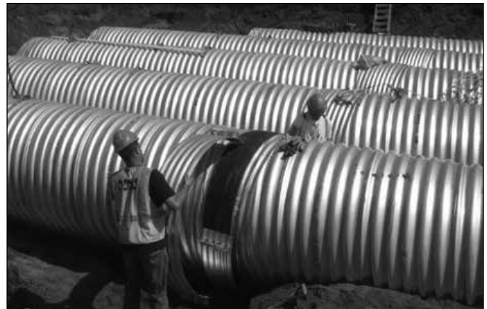
Installation of corrugated band with flat neoprene gasket
