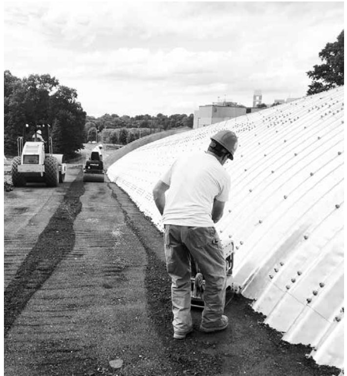
Figure 7. Adequate, uniform compaction is critical to building soil/aluminum structures.
