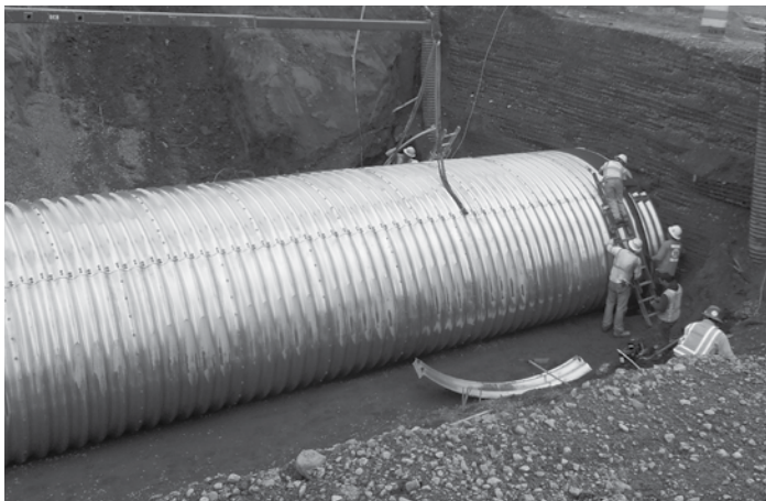
Completing the Final Ring
