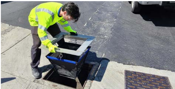
Filters can be maintained by a vac truck or by hand.
