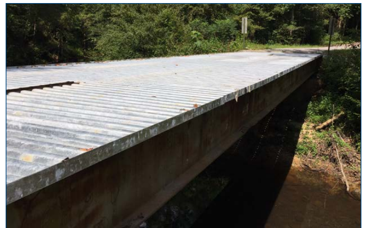
A continuous bridge deck
