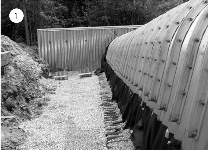
Loosely placed geotextile over scallop plate and exterior of invert plate.
