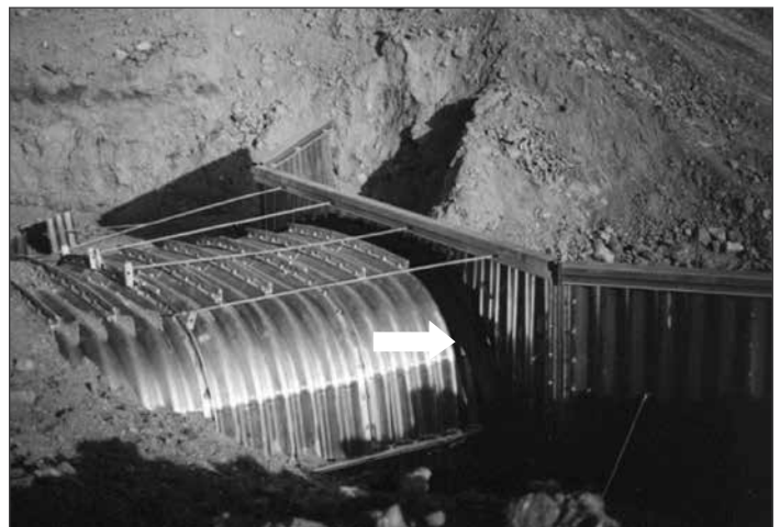
Once the headwall is installed, install fabric behind the headwall where any gapping occurs.
