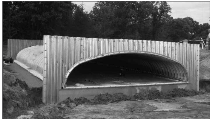
Proper installation of toewall when invert and headwall are utilized.
