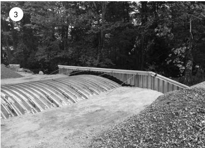
Granular material placed in balanced manner.
