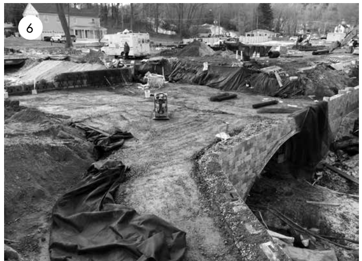
Compact material with a vibratory plate compactor.
