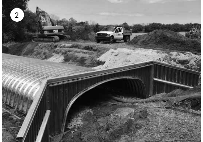
Backfill material is placed carefully before 8" lifts are spread evenly and compacted.
