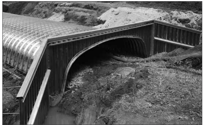
ALBC with headwall and wingwalls.
