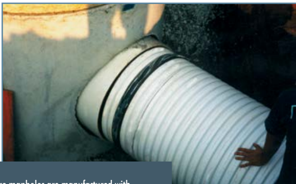
Use a Contech manhole gasket for 12"-36" A-2000. For 8" - and 10" - diameter pipe, use a standard A-2000 double sealing gasket.
