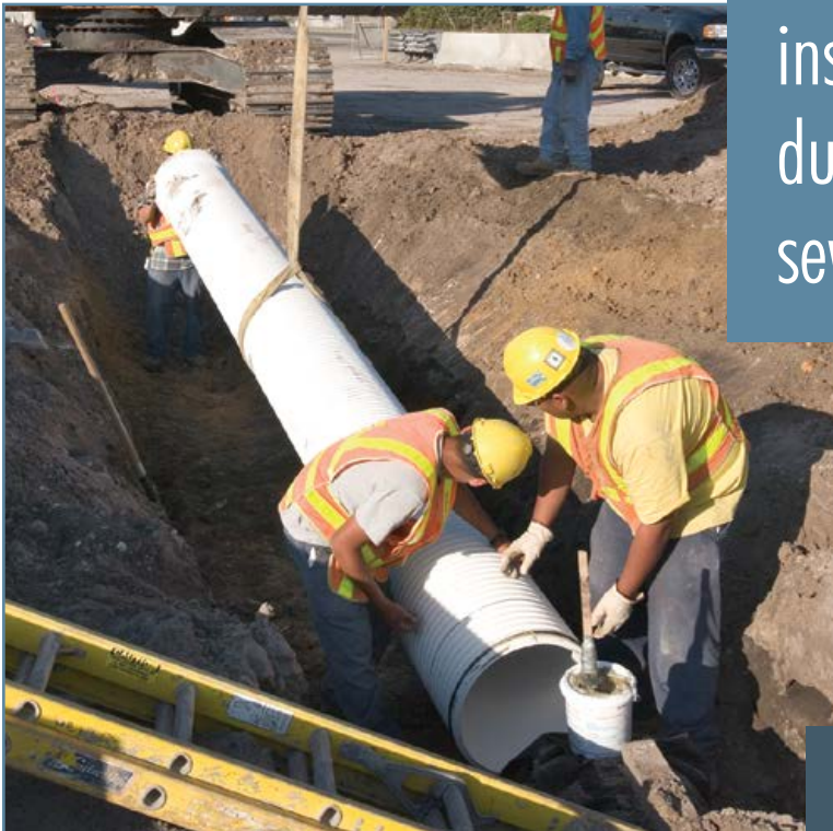
A-2000's unique gasketed joint design allows easier field assembly. Pipe diameters of 4"-18" can be joined by hand, without the use of mechanical equipment.
