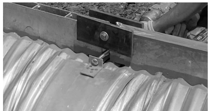
Temporary or permanent steel closure plates can be used to help align the grate. These can be bolted on or clamped across the gap. Other means of alignment include prybars and wooden tiedowns.
