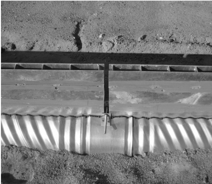
Slotted Drain™ System with modified HUGGER® band.
