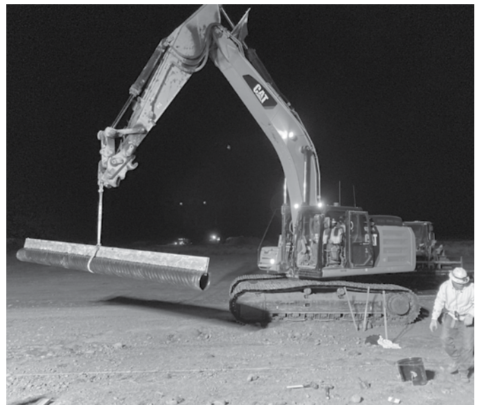
Lifting Polymer Coated Steel Slotted Drain™ System with nylon slings at a project site.
