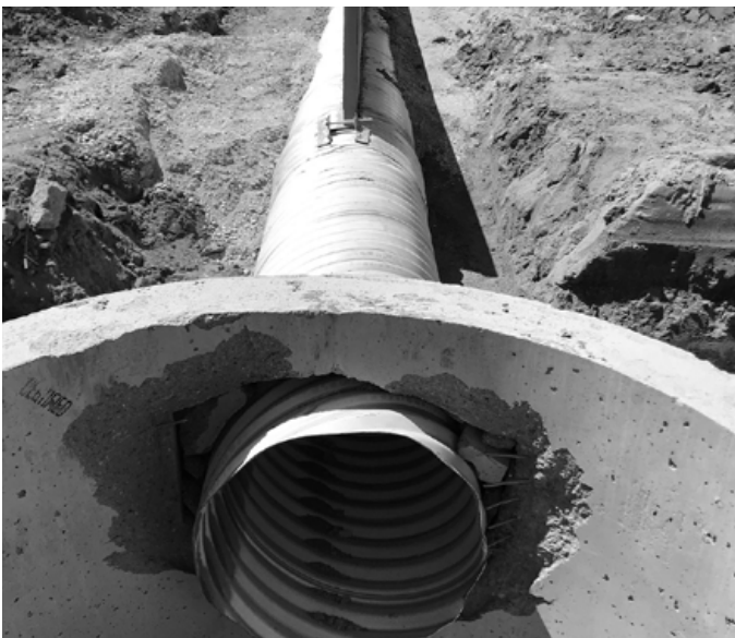
Slotted Drain System connected to a corrugated steel pipe inserted into a concrete manhole.
