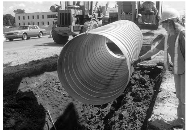
Reduced excavation due to the smaller outside diameter of ULTRA FLO®.
