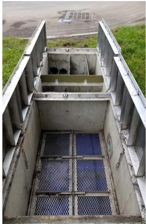
*The Water Polisher is accessible and can be maintained from the finish surface.*
