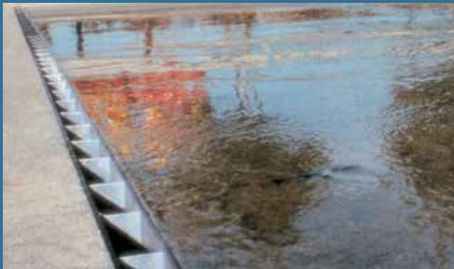
Slotted Drain is widely used in parking areas and driveways, where its ability to provide efficient drainage, without the need for hazardous dips in pavement, is a safety asset.
