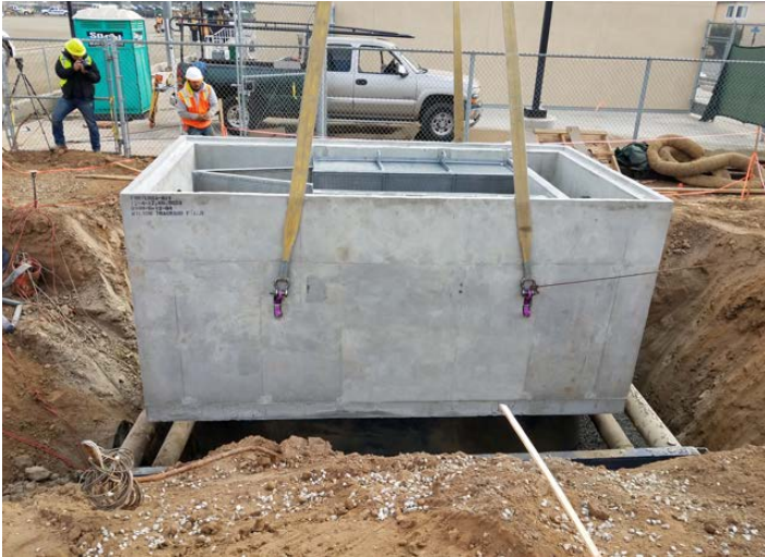
Minimum excavation is required and the unit is delivered in with a bottom and top slab to minimize weight.
