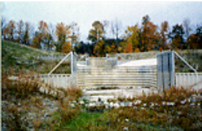
Installing aluminum drop structures permitted grade reductions, halting damaging erosion.
