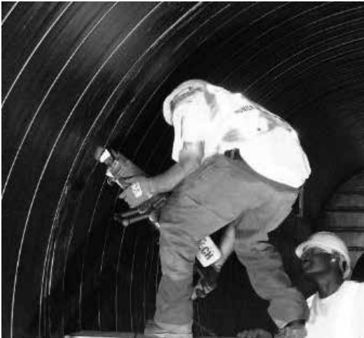
Internally welding pipe joints. The pipe needs to be backfilled prior to the joints being welded together. The pipe should be clean and dry. The gap between the two pipes should be limited to 1.5" maximum. The maximum pipe misalignment is 1/4". Pipe joints outside recommendations could result in higher joint welding costs.
