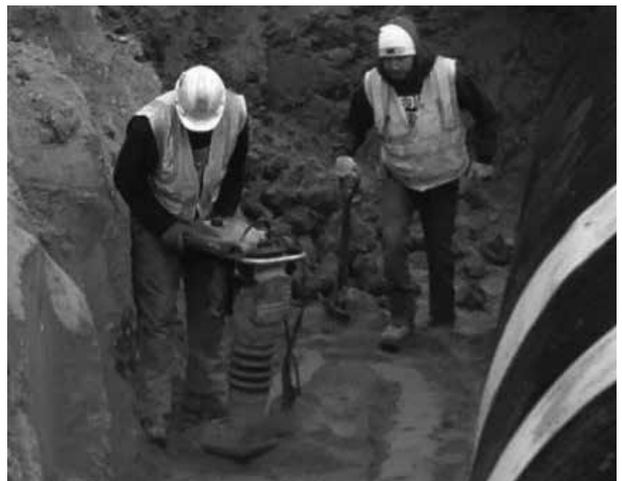
Compaction with vibratory equipment.
