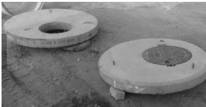
Precast option for manhole riser caps.
