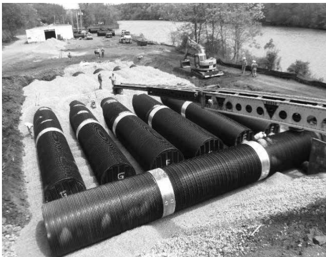
Placing backfill with a stone conveyor.
