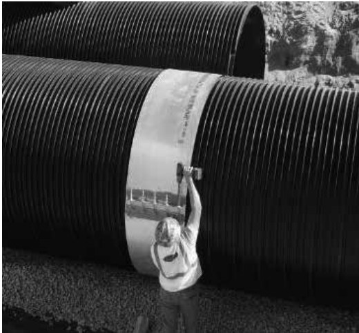
Tightening bolts on a flat band.
