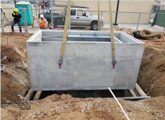
Minimum excavation is required and the unit is delivered in base and top sections that join together.
