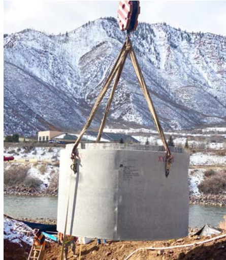
Step 2: Lift and place middle riser.
