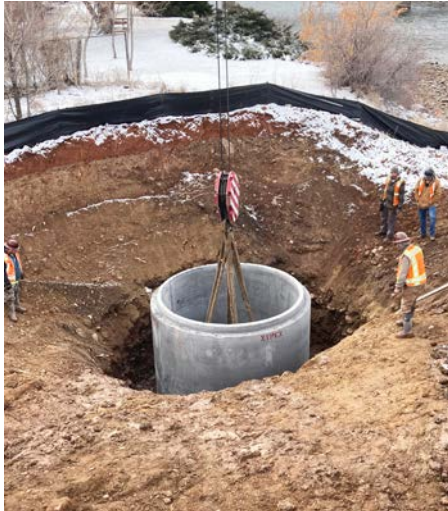
Step 1: Install the base section.
