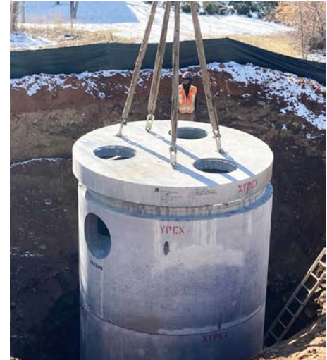
Step 3: Place top slab with access holes.
