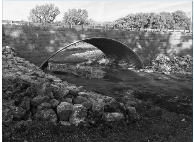
BridgeCor External Rib System after construction
