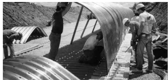
Assembly of ALBC Shell onto Full Invert
