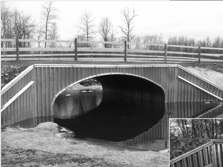
Aluminum Box Culvert Stream Crossing
