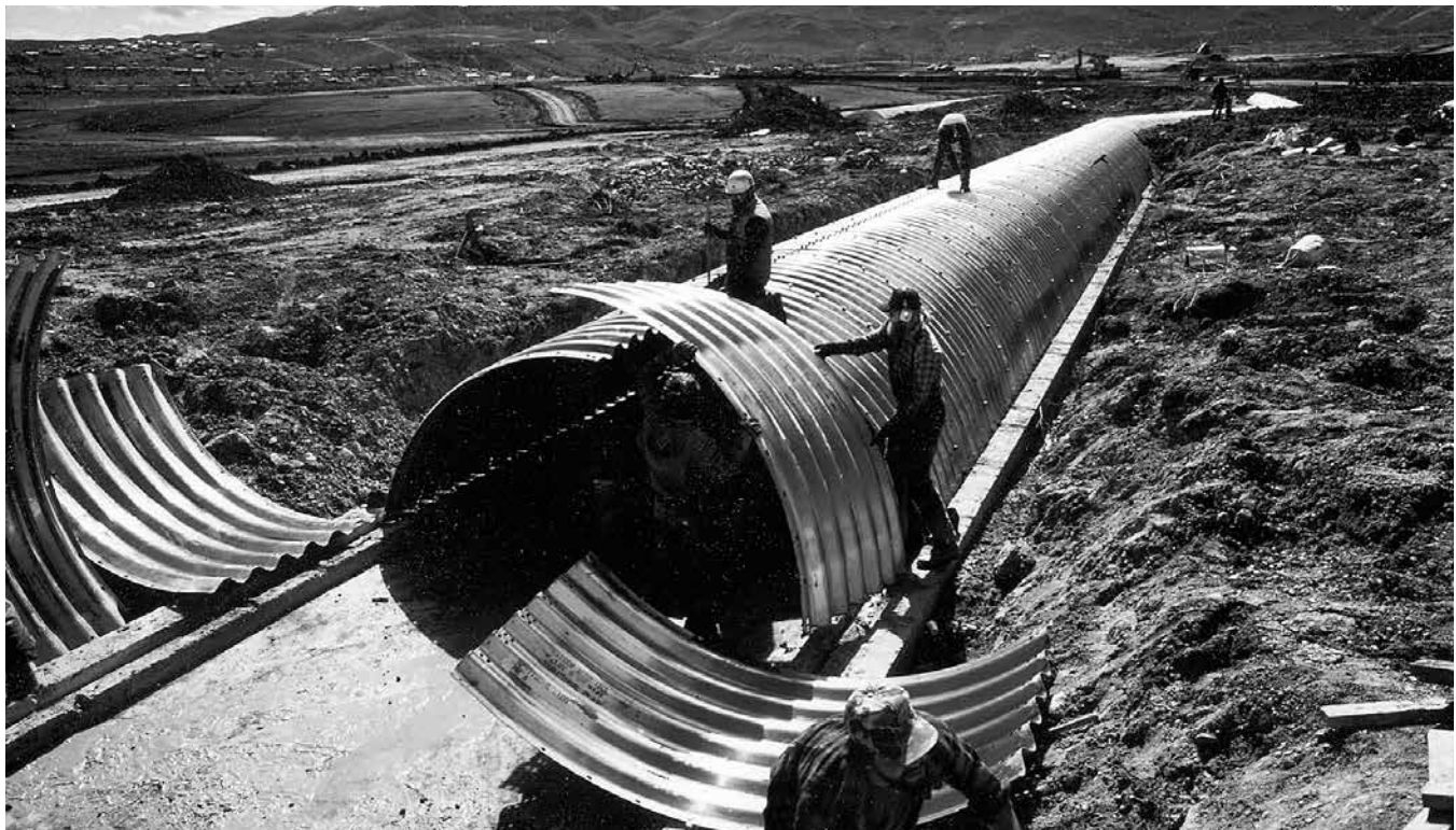
Assembly of Aluminum Structural Plate Single Radius Arch
