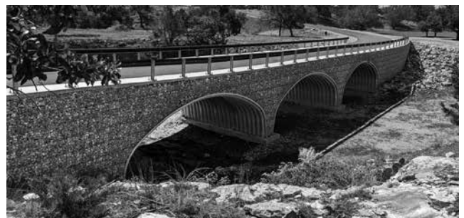
BridgeCor with Vist-A-Wall Welded Wire Wall System in Harper, TX.
