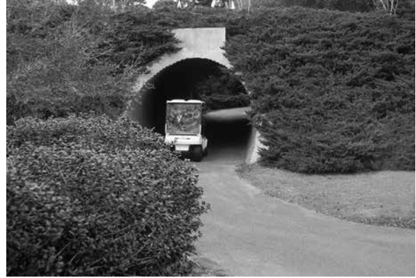
MULTI-PLATE Golf Cart Underpass
