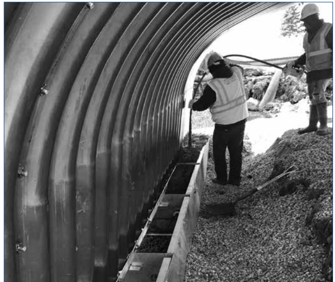
Pre-assembled plate structure can be set on footers
