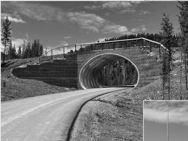
BridgeCor with a Vist-A-Wall Welded Wire Wall System for a Private Development
