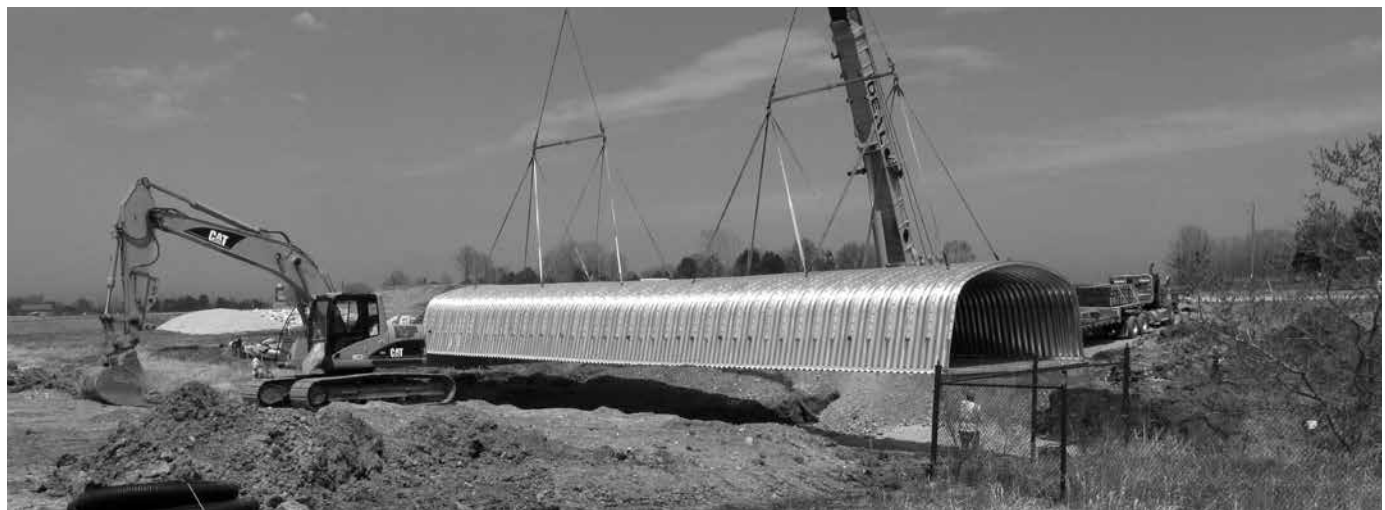
Fully Assembled Aluminum Box Culvert Being Set in Place
