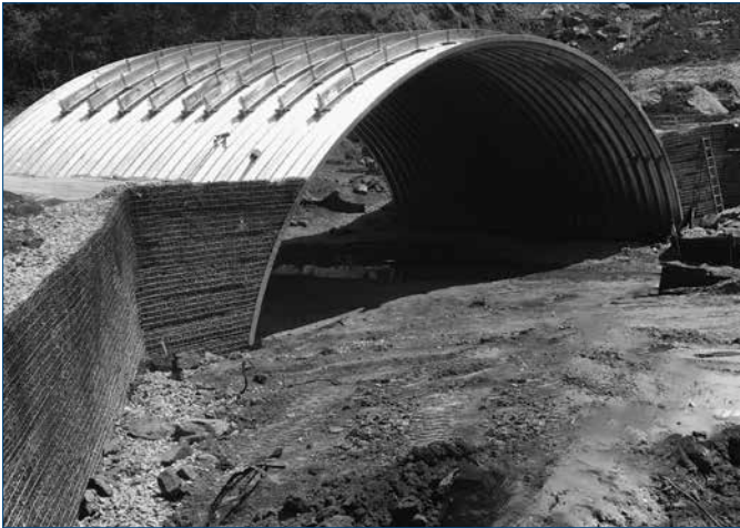
BridgeCor (64'-2" x 19'-7") External Rib System with Vist-A-Wall Welded Wire Wall System during construction
