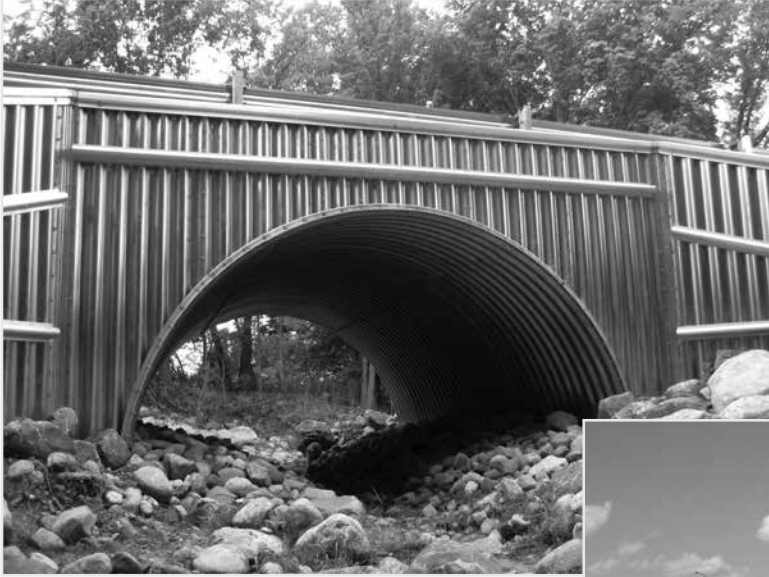
Aluminum Structural Plate Stream Crossing
