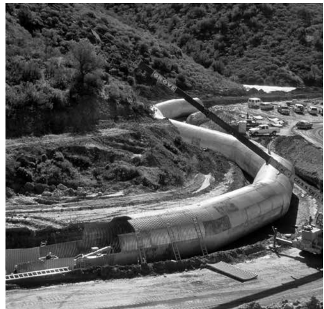
Along the Eastern Transportation Corridor in Orange County, California, this Key-Hole Slot MULTI-PLATE® structure was designed for the 115 ft. of cover.
