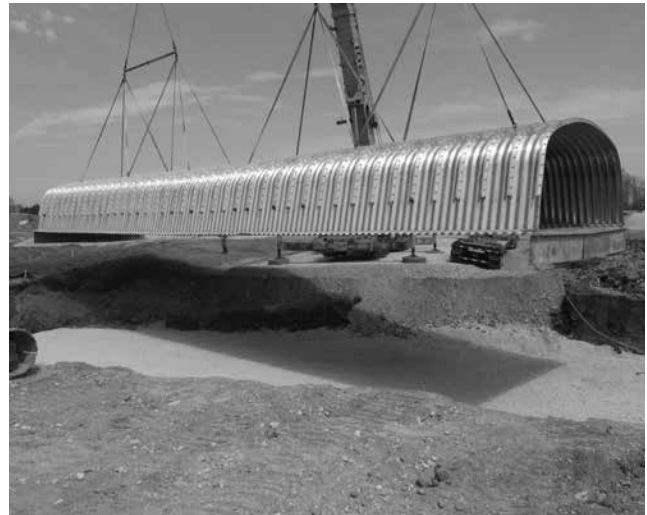
Aluminum Box Culvert installation
