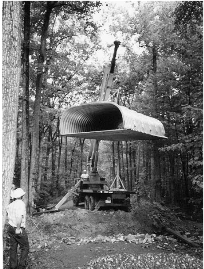
Lifting of Aluminum Box Culvert
