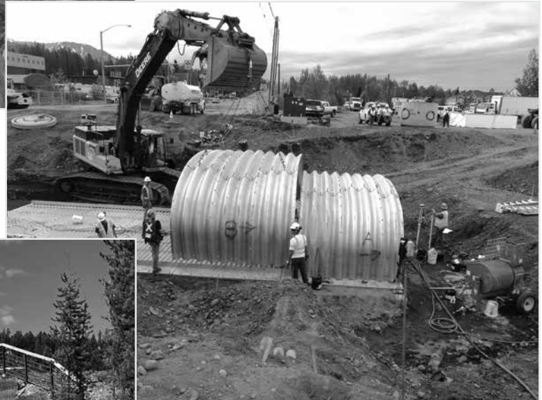
BridgeCor Box Culvert Assembly
