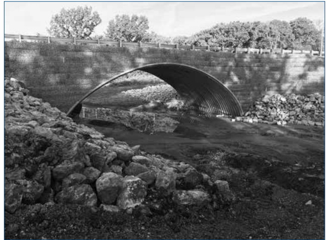
BridgeCor External Rib System after construction
