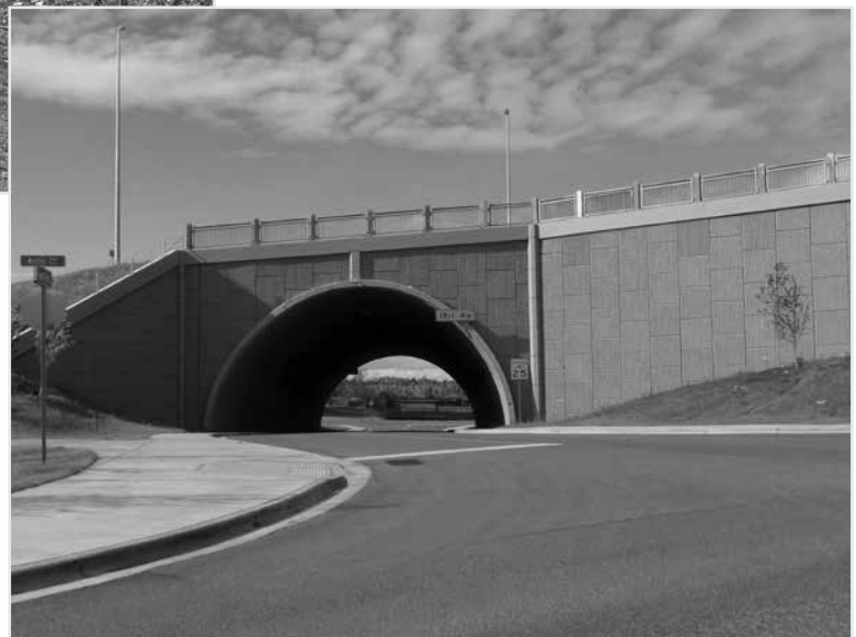
BridgeCor with a MSE Precast Panel Wall System on a DOT Project
