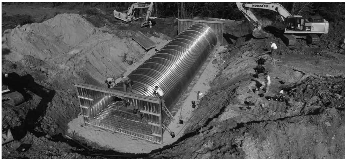
Assembly of Aluminum Structural Plate with Headwalls
