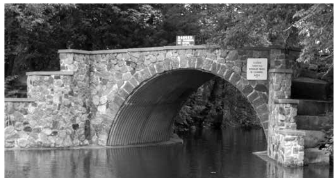
At the time of inspection in 2012, this Steel Structural Plate Single Radius Arch was 72-years-old. Installed c. 1940 | Inspected in 2012
