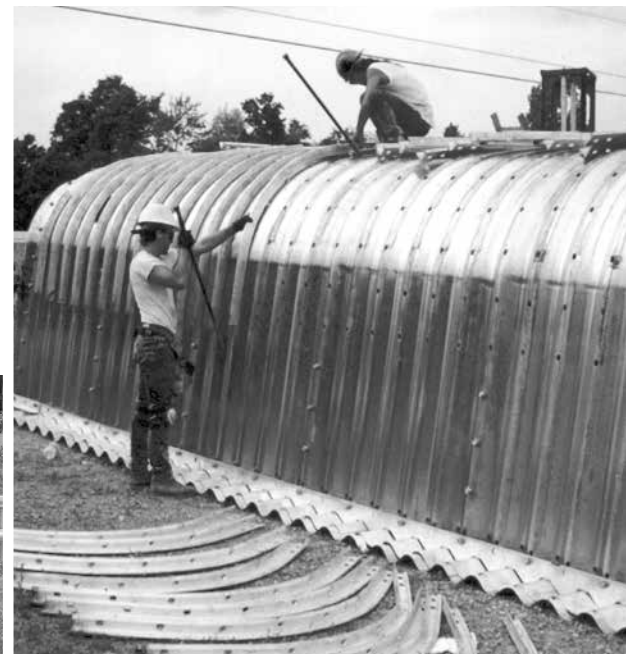
Installation of Ribs
