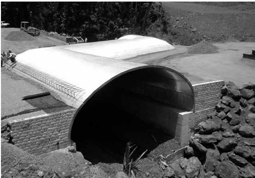
High-profile arch SUPER-SPAN in Puerto Rico spanning a wetland and providing a wildlife crossing
