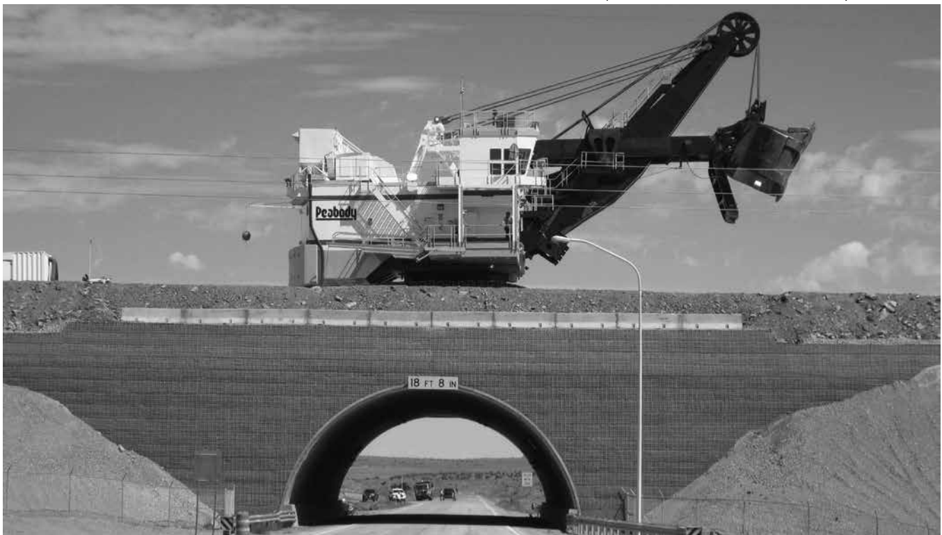
BridgeCor® with Vist-A-Wall Welded Wire Wall System at Peabody Coal Mine near Grants, New Mexico.
