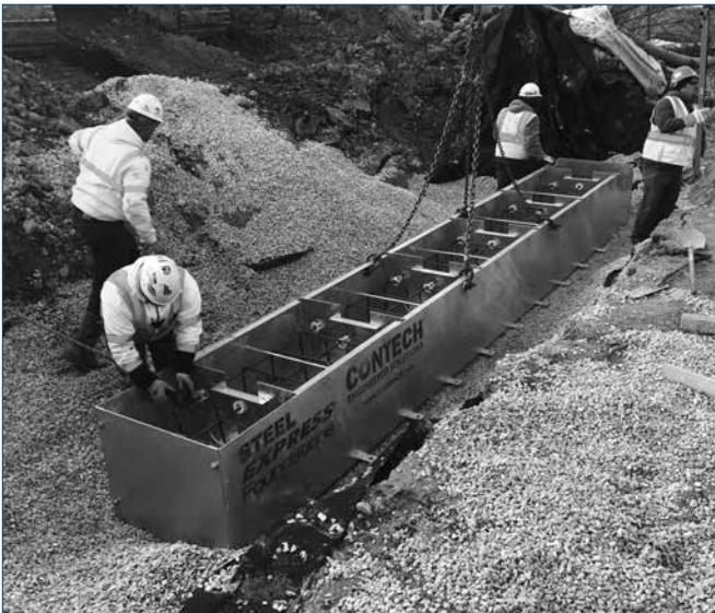
Set footers in place
