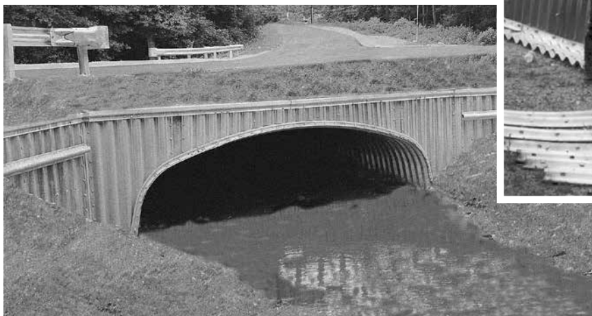
Corrugated Aluminum Box Culvert with Headwall Package
