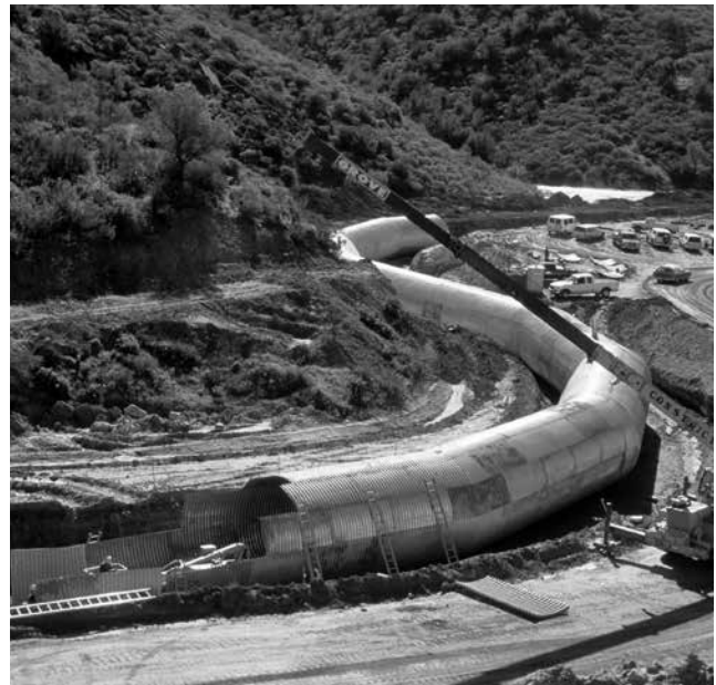
Along the Eastern Transportation Corridor in Orange County, California, this Key-Hole Slot MULTI-PLATE® structure was designed for the 115 ft. of cover.
