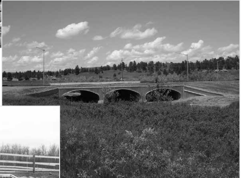
Aluminum Box Culvert Triple Span
