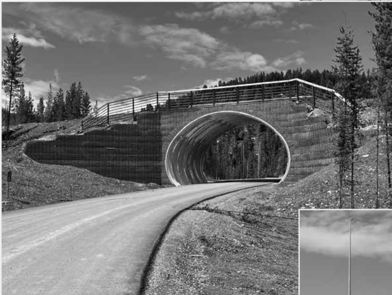
BridgeCor with a Vist-A-Wall Welded Wire Wall System for a Private Development
