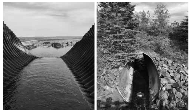
Bay of Fundy | Robinston, ME 52-Year-Old Aluminum Structural Plate Installed in 1966 | Inspected in 2018
