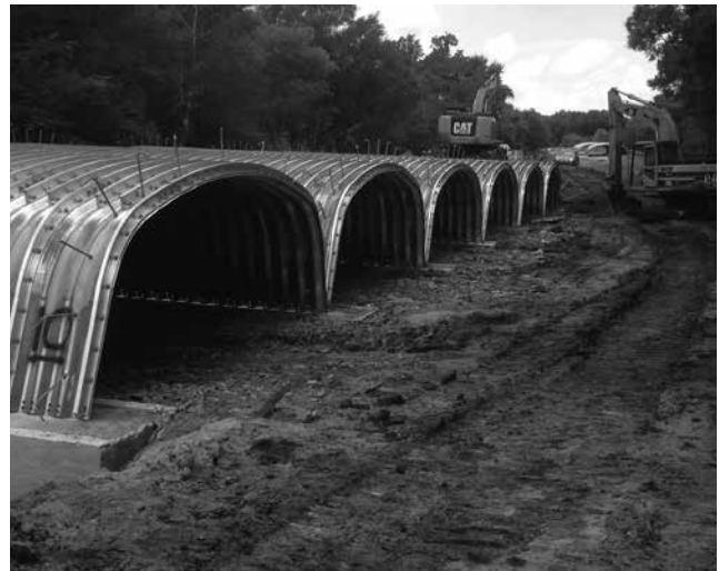
Aluminum Box Culvert multi-cell installation
