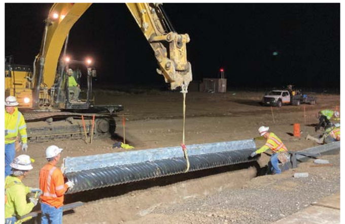
Slotted Drain™ surface runoff collection system is ideal for aprons, runways, taxiways and deicing areas.
