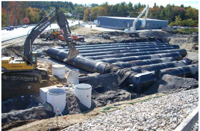
CMP Detention System provides the perfect solution for FAA's requirements to remove any ponded water adjacent to a runway.
