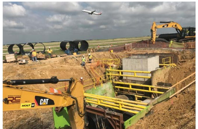
DuroMaxx® SRPE is an extremely efficient solution for glycol storage able to handle the heavy live-loading of an Airbus A380.
