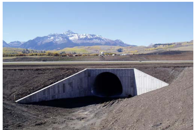
Structural Plate offers a wide range of shapes and sizes for specific site considerations and deep cover applications
