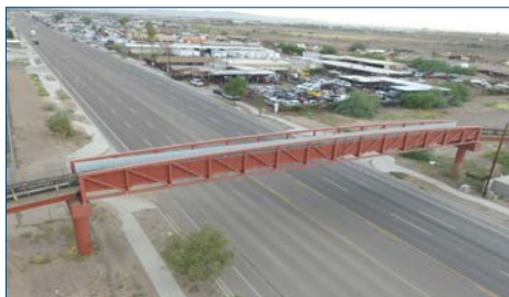
Continental Capstone® Conveyor Phoenix, AZ
