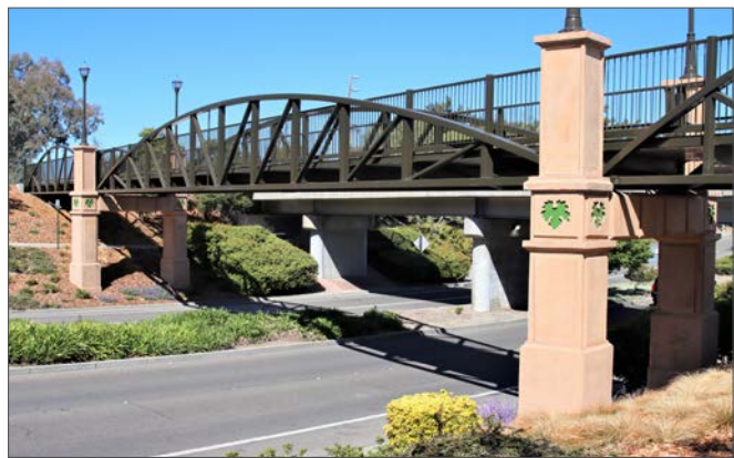
Continental Pedestrian Truss Bridge
