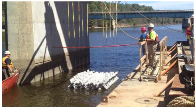
Bundled Option - No Dewatering Required
