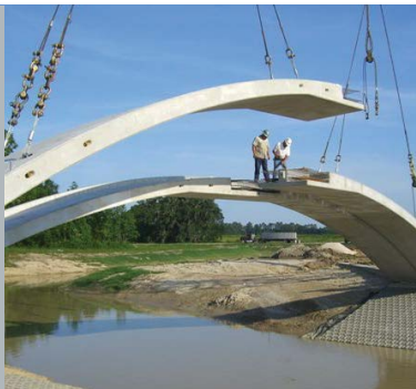
TWIN LEAF CONSTRUCTION
