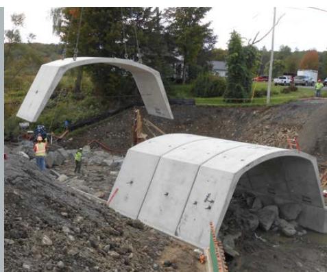
PRECAST ARCH UNITS
