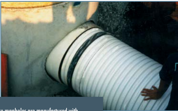
Use a Contech manhole gasket for 12"-36" A-2000. For 8" - and 10" - diameter pipe, use a standard A-2000 double sealing gasket.
