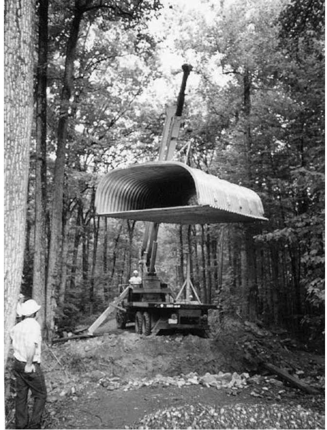
Lifting of Aluminum Box Culvert
