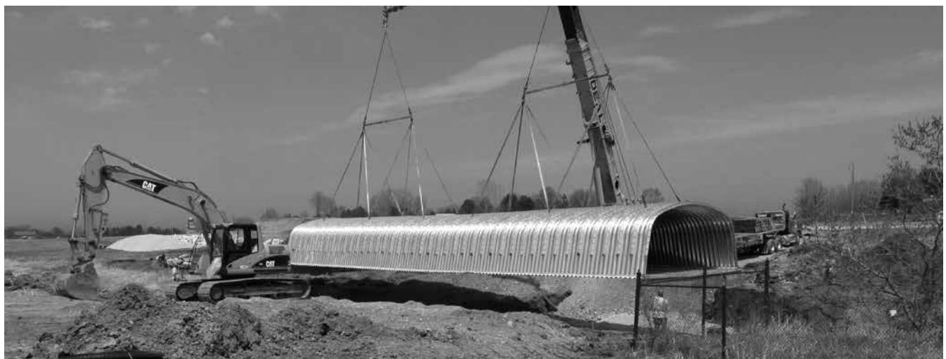
Fully Assembled Aluminum Box Culvert Being Set in Place
