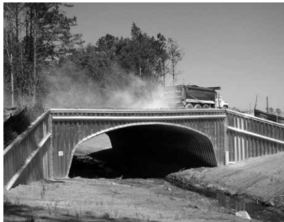
Aluminum Box Culvert with Full Aluminum Headwall Package
