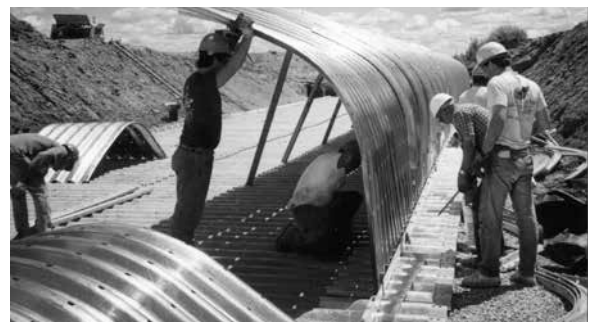
Assembly of ALBC Shell onto Full Invert
