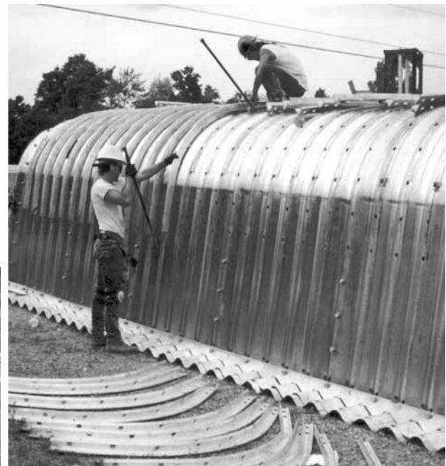
Installation of Ribs
